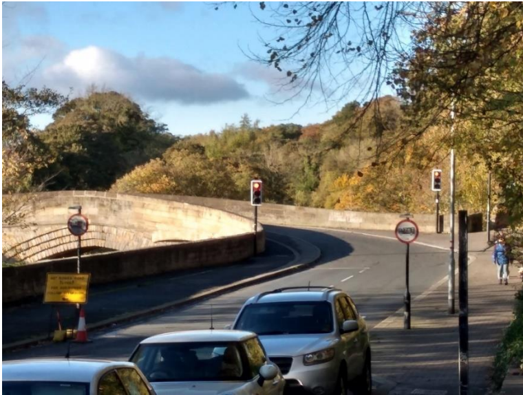
Fig. 11 View of the County Bridge from Bridgegate
