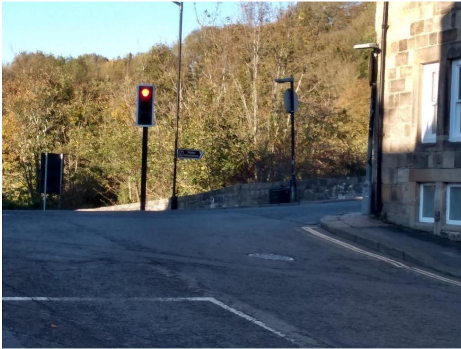
Fig. 9 Turn from B6277 onto the County Bridge
