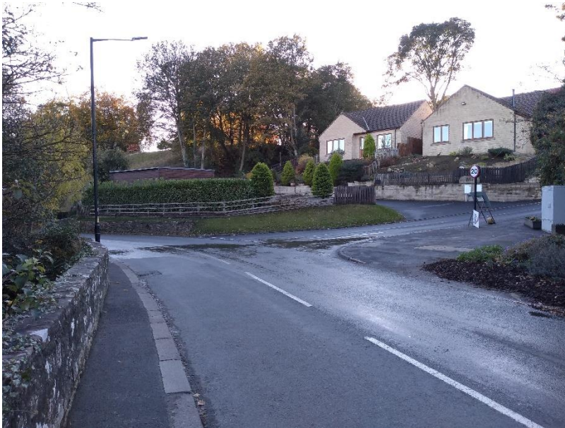
Fig. 5 Junction of B6277 and Gill Lane
